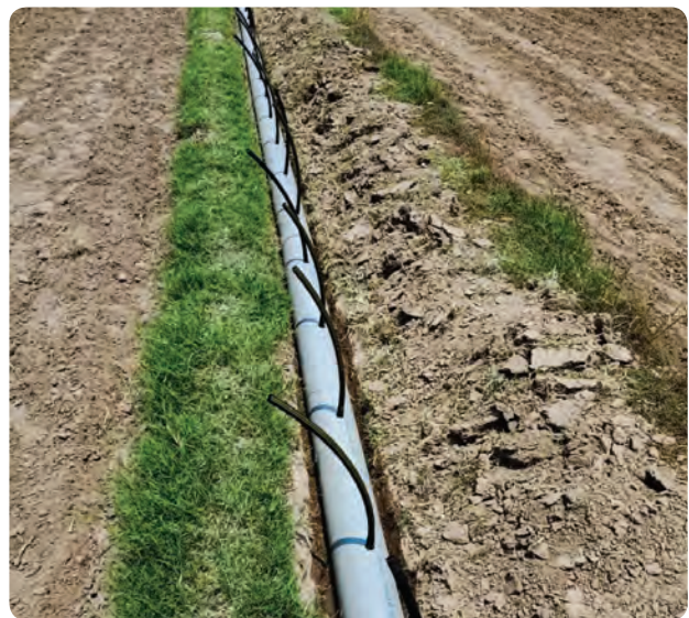
Laying of Submain. L/L spacing 0.6m
